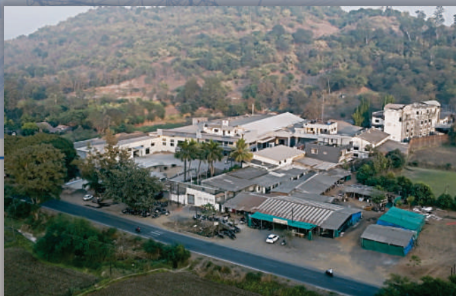
HEX - BCA factory at Vapi, Gujarat
